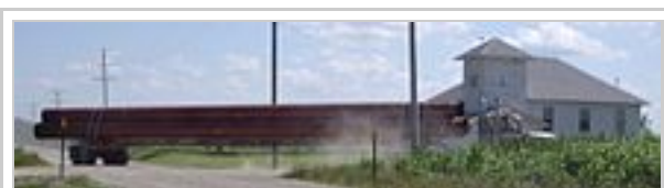
Truck hauling 36-inch pipe to build Keystone-Cushing pipeline (phase 2) southeast of Peabody, Kansas (2010)
